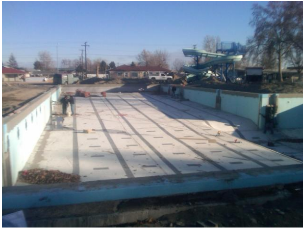
The Memorial Pool "Before" and during Construction
