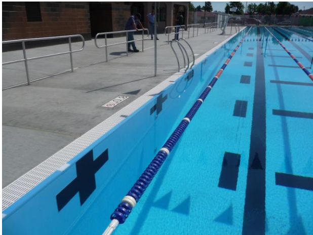
The newly installed Myrtha® gutter system.
